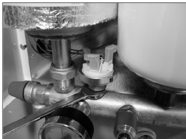
FIG. 23 - PRESSURE SWITCH
