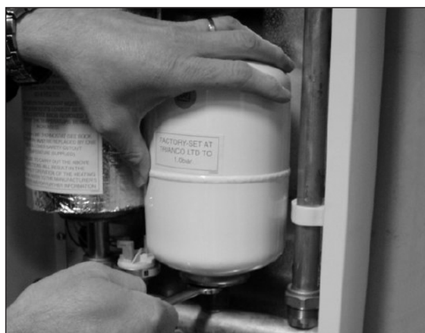
FIG. 24 - EXPANSION VESSEL
