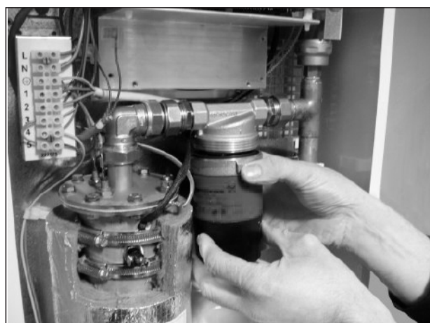
FIG. 25 - PUMP HEAD
