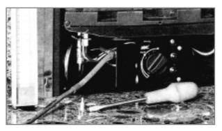
If the setting pressure is too low, but the meter pressure is acceptable, then a problem in the supply pipework is to be suspected. This will be dirt and debris, kinked or inadequate size pipes, restriction in a fitting or solder flashing across a joint.
