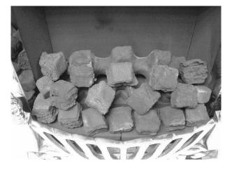
g) Select the remaining four coals and position to fill the gaps left at the top rear of the fuelbed. The coals will locate naturally into the depressions in the top rear of the fuelbed. See below fig. 17 below.
