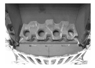
Select seven of the coals and arrange along the front ceramic coal support using the shallow depressions as guidance for the coal position. See fig. 14 below
