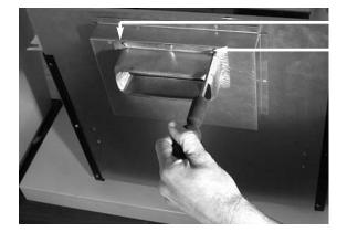
4 off Flue Spigot Fixing screws
