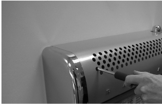
Fig. 8 Removing the Upper Outer Case Fixing Screws
