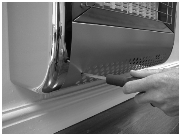
Fig. 4 Remove the Lower Outer Case Fixing Screws
