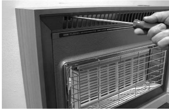
Fig. 8 Removing the Upper Outer Case Fixing Screws
