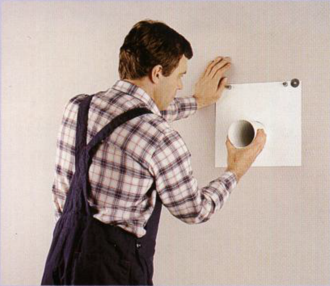
Step 3. Fit boiler mounting plate.
