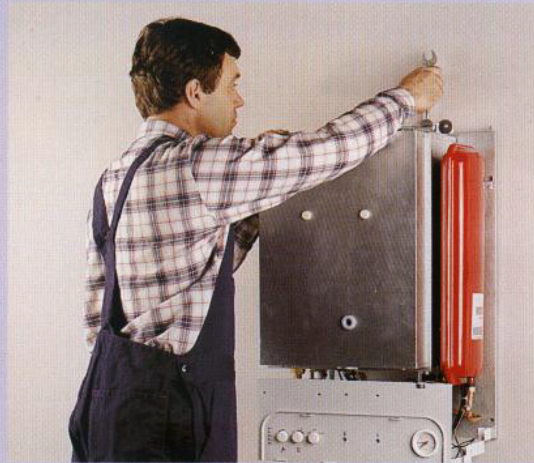
Step 4. Fit boiler to mounting plate.
