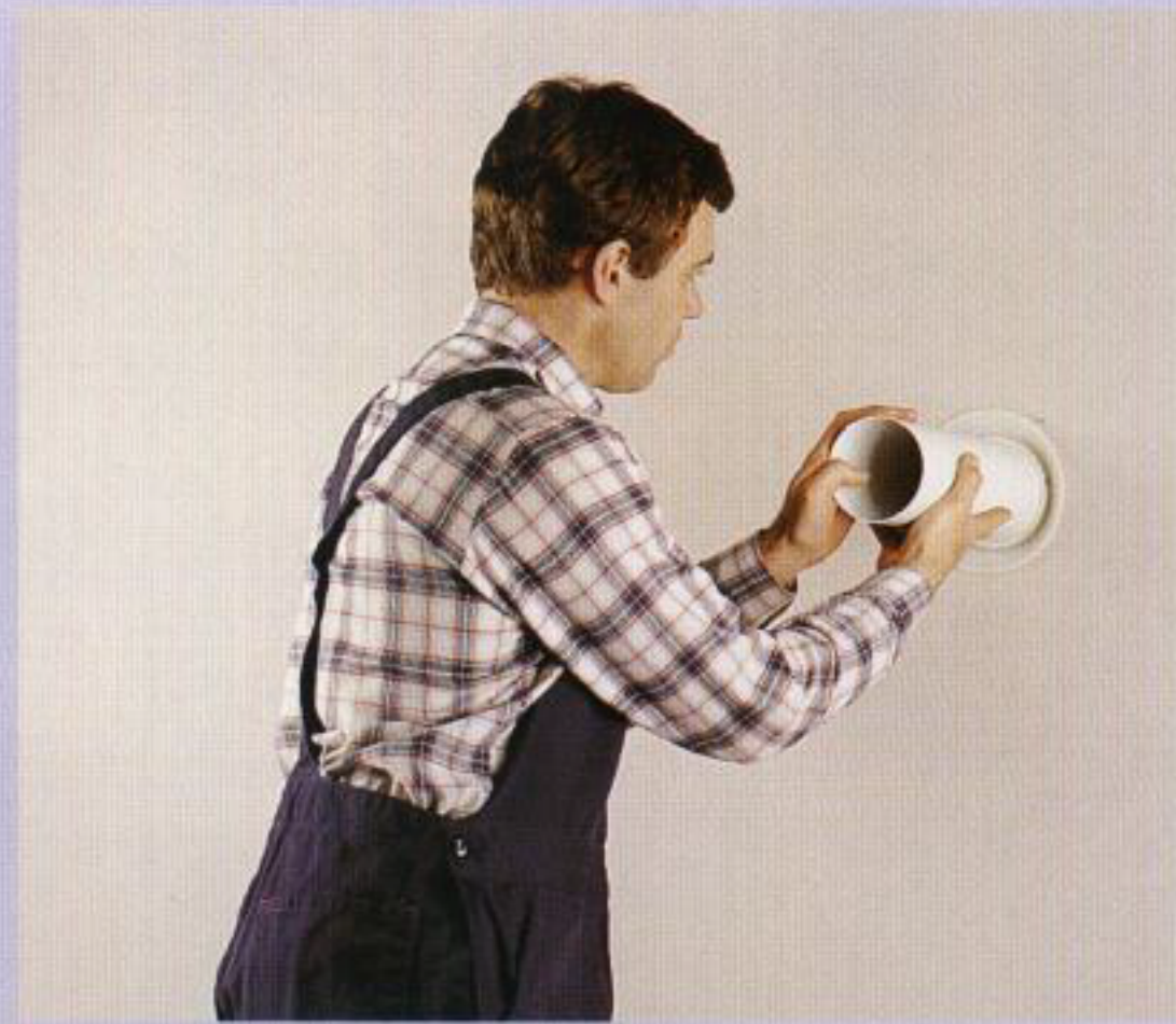
Step 2. Slide flue, with terminal fitted, into position.
