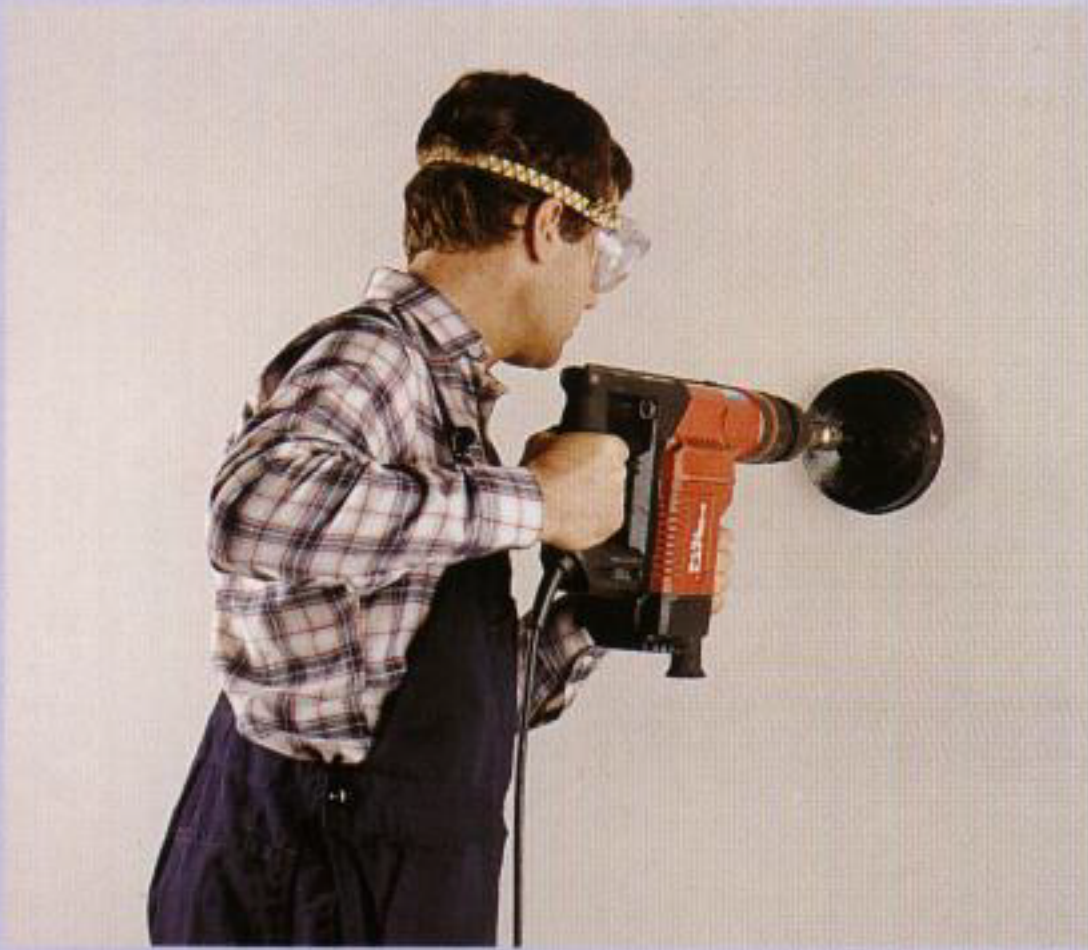
Step 1. Drill flue hole.
