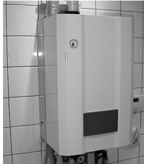
Figure 8 EC25 Solar Compatible Condensing Boiler
