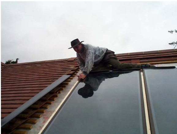
Figure 25 Fixing flashing rails
