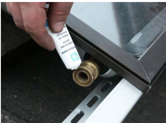
Figure 44 Silicone in connector socket
