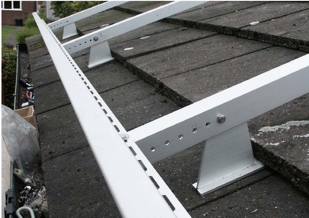
Figure 37 Frame support detail
