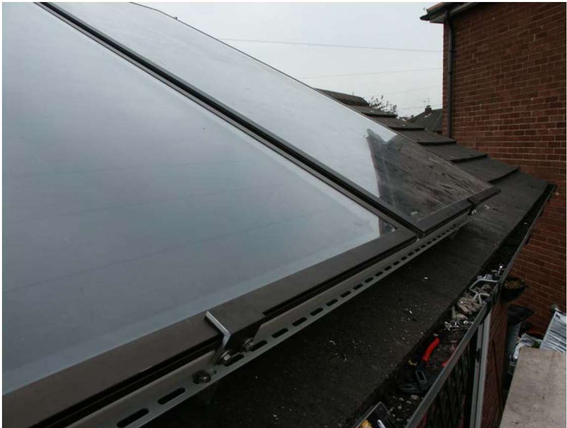
Figure 50 Panels clamped to frame.
