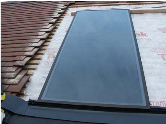
Figure 12 Positioning panel
