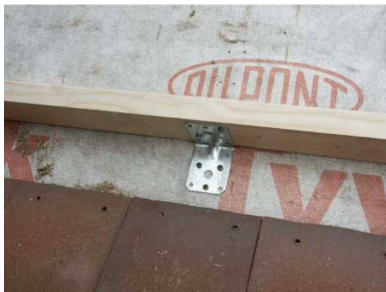
Figure 4 Fixing Bottom Rail
