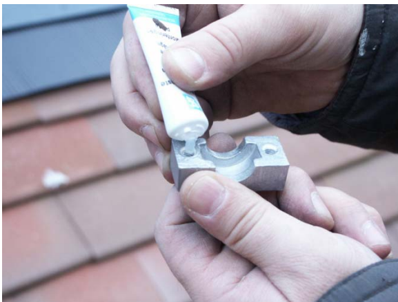
Figure 16 Jointing clamp
