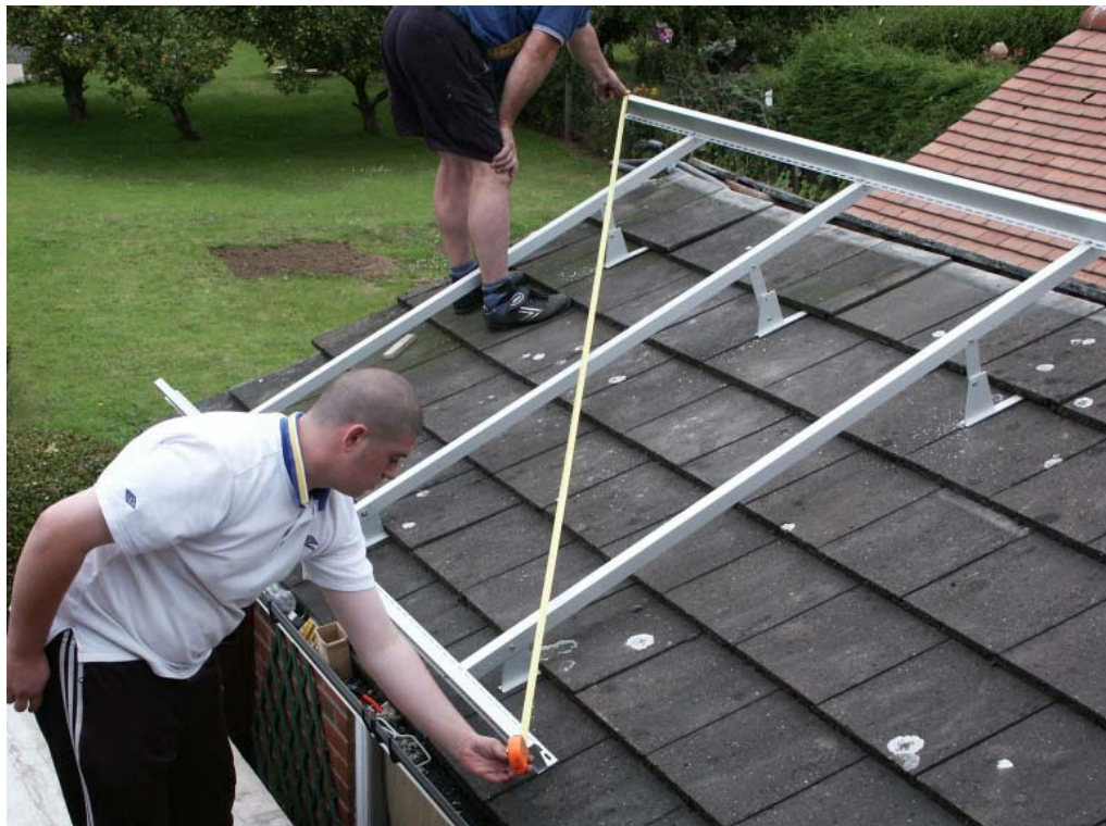
Figure 40 Checking frame dimensions
