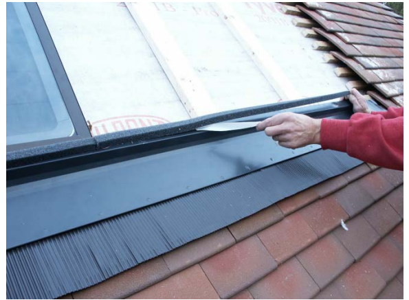
Figure 13 Fixing foam strip
