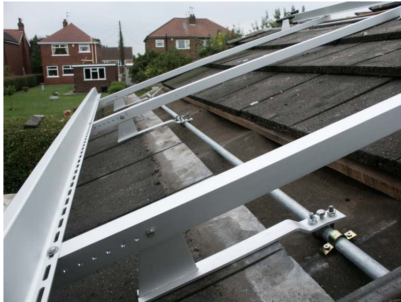
Figure 41 Frame fixed to roof
