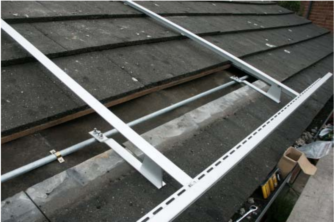
Figure 39 Roof tile removal
