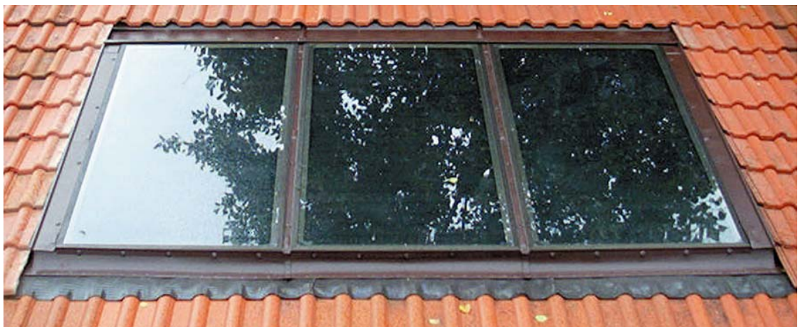
Figure 54 In roof 3 panel flashing and mounting frame
