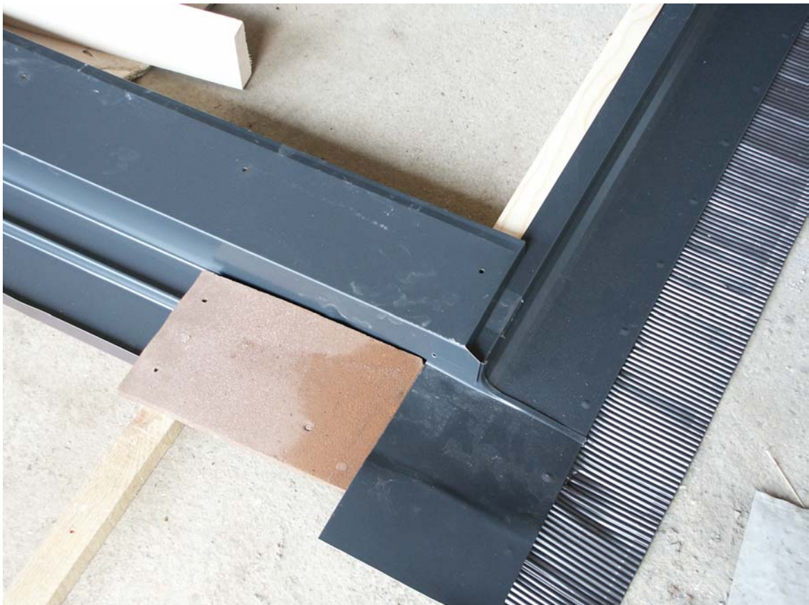
Figure 3 Checking roof tile alignment
