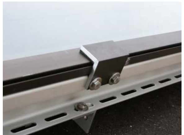
Figure 49 Panel clamp
