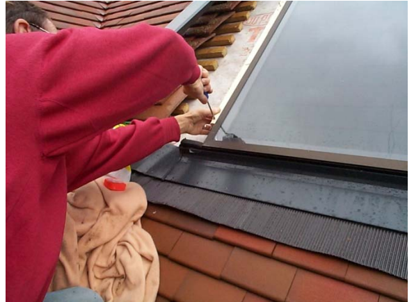
Figure 22 Fixing edge timber flashing rails
