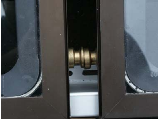
Figure 46 Panel socket and spigot
