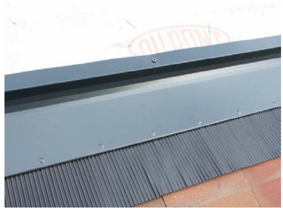
Figure 8 Fixing apron flashing
