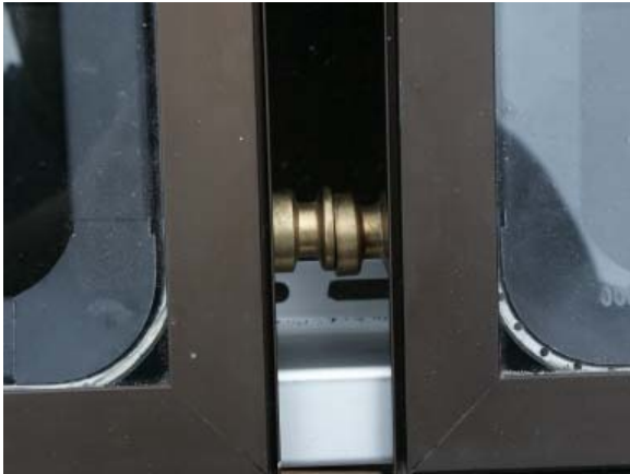
Figure 16 Jointing clamp
