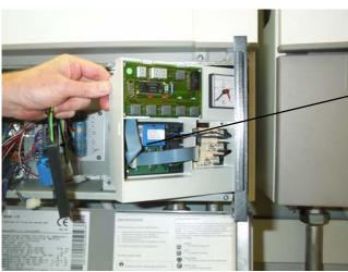
Open the R/H door and front smoked grey panel to reveal both sides of the standard interface. Shown here in the bottom L/H corner
