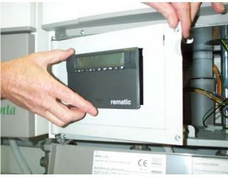
Place 2945 C3 K *rematic*® control in opening and remove the control cover plate (press down and in the direction of the arrow)
