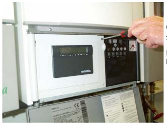
Close both doors and secure with the 2 existing screws.
