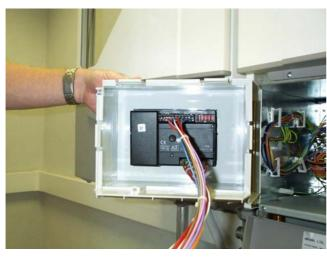
From the wiring harness insert the 4 plugs (two black, one green and one grey) into positions P3, P2, P11 and P12 in the back of the 2945 C3 K *rematic*® control unit.
