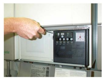
Drop down lower (grey) cover and remove the two securing screws from the left hand door.
