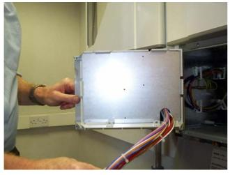
Replace the steel closing plate in the back of the door (taking care that the wires are located in the cut out)
