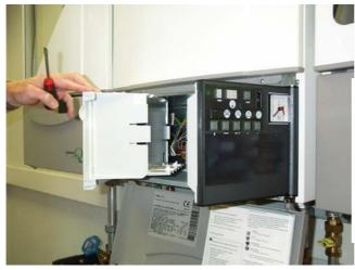
Open both doors to reveal main electrical compartment and site wiring connections.
