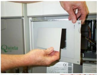
Remove the plastic cover from the front of the left hand door (push free from the back)
