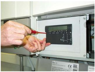
Secure the control using the two locking screws (quarter turn latches) located just below the display on the left and right hand sides as shown
