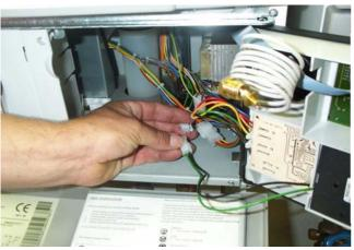
Plug *rematic*® interface cables into mating boiler plugs as follows.
