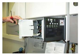
Open both doors to reveal main electrical compartment and site wiring connections.
