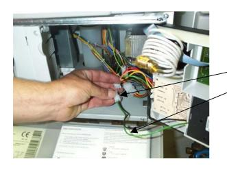
Disconnect the 0-10v interface from the boiler wiring (plug X19) and unplug the ribbon cable. Coil up the loose cable and tape it to the back of the interface module to keep it clear of the door.
