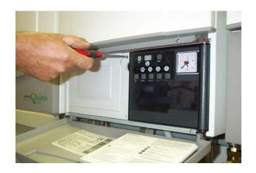
Drop down lower (grey) cover and remove the two securing screws from the left hand door. (retain for re-securing)
