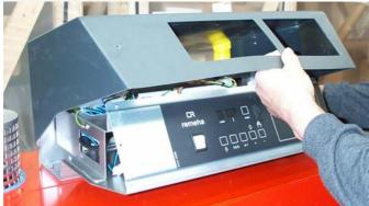
Release the 4 control panel cover screws and remove the cover
