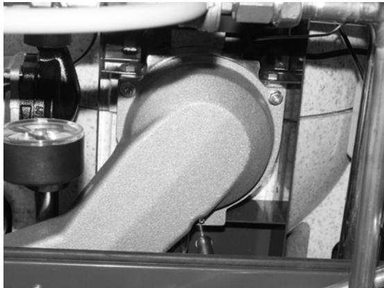
Figure 32: Flue baffle
