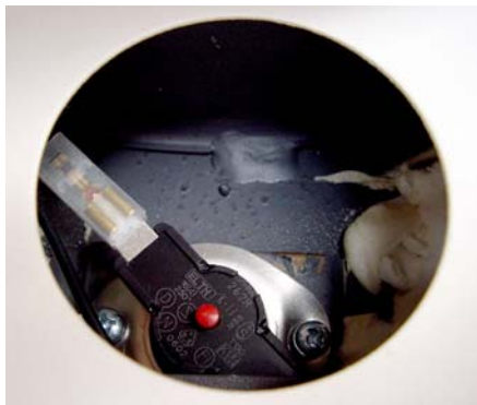
Fig. 22: Safety thermostat reset button
